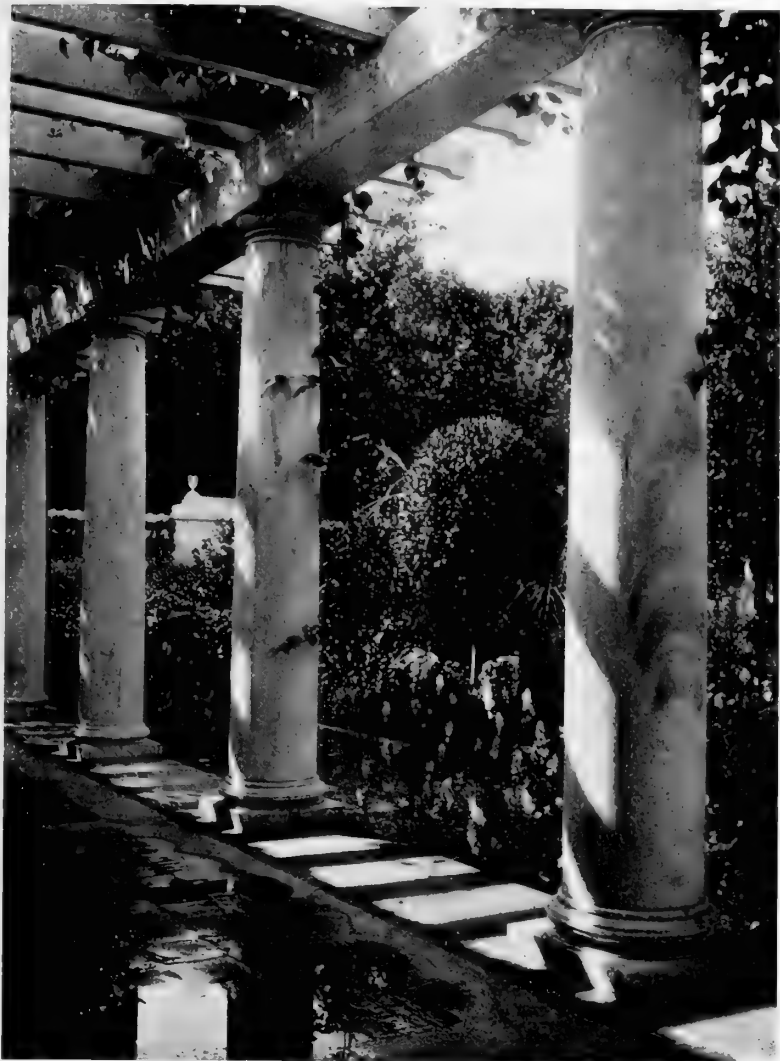
Looking Through the Pergola
